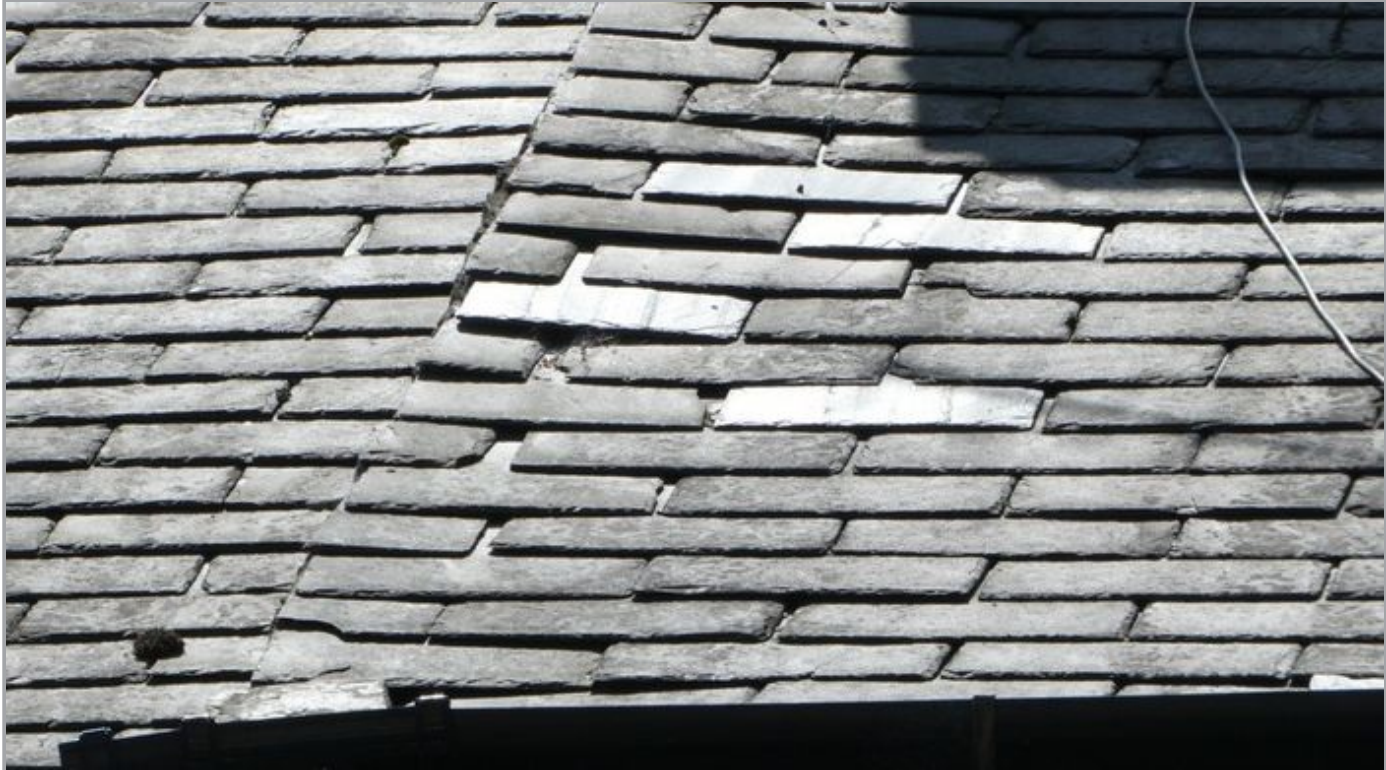
Lifted/Loose/Damaged Coverings
