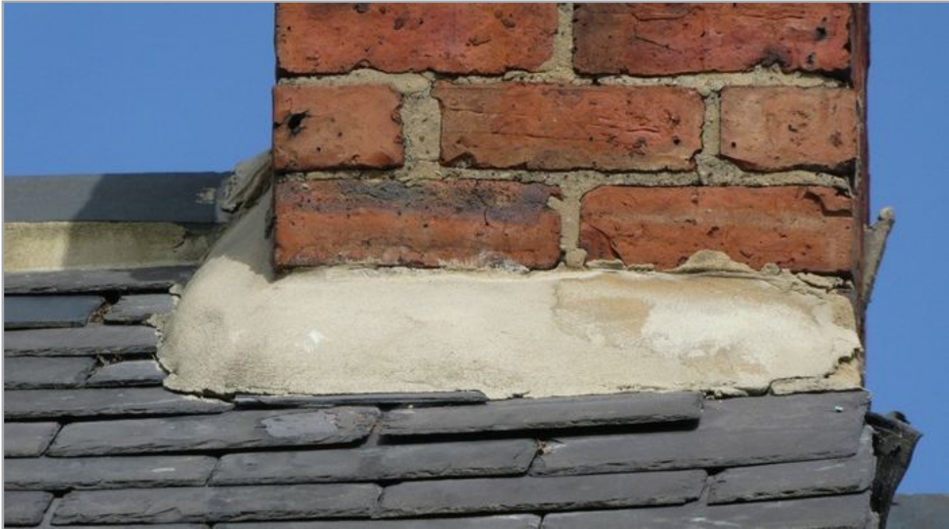
Inadequate Flashing
