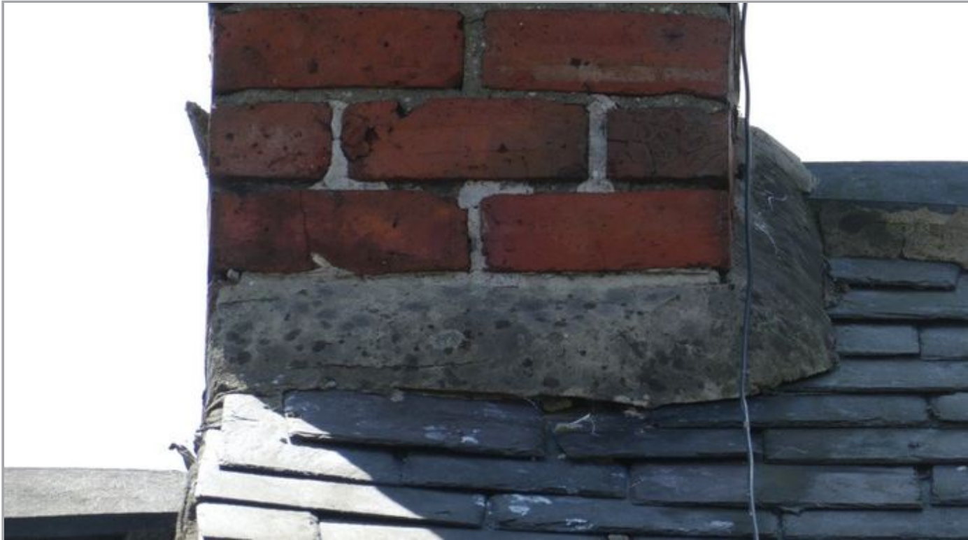
Inadequate Flashing
