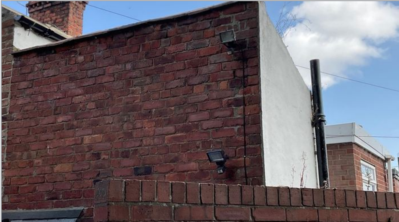
Solid Construction Limited Insulation
