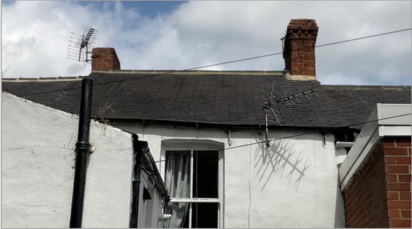
Misaligned Guttering
