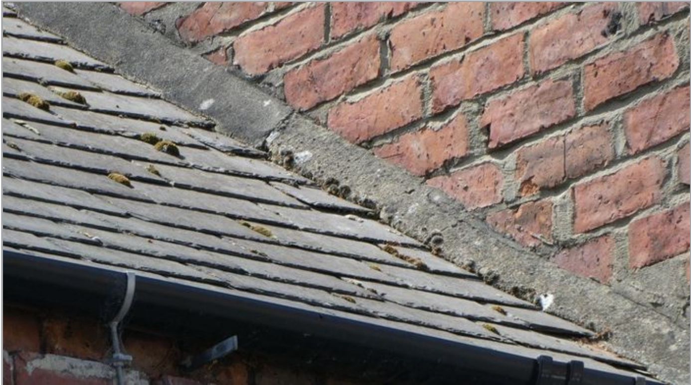
Inadequate Flashing
