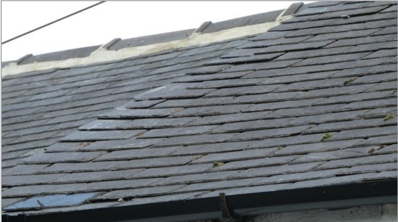
Lifted/Loose/Damaged Coverings
