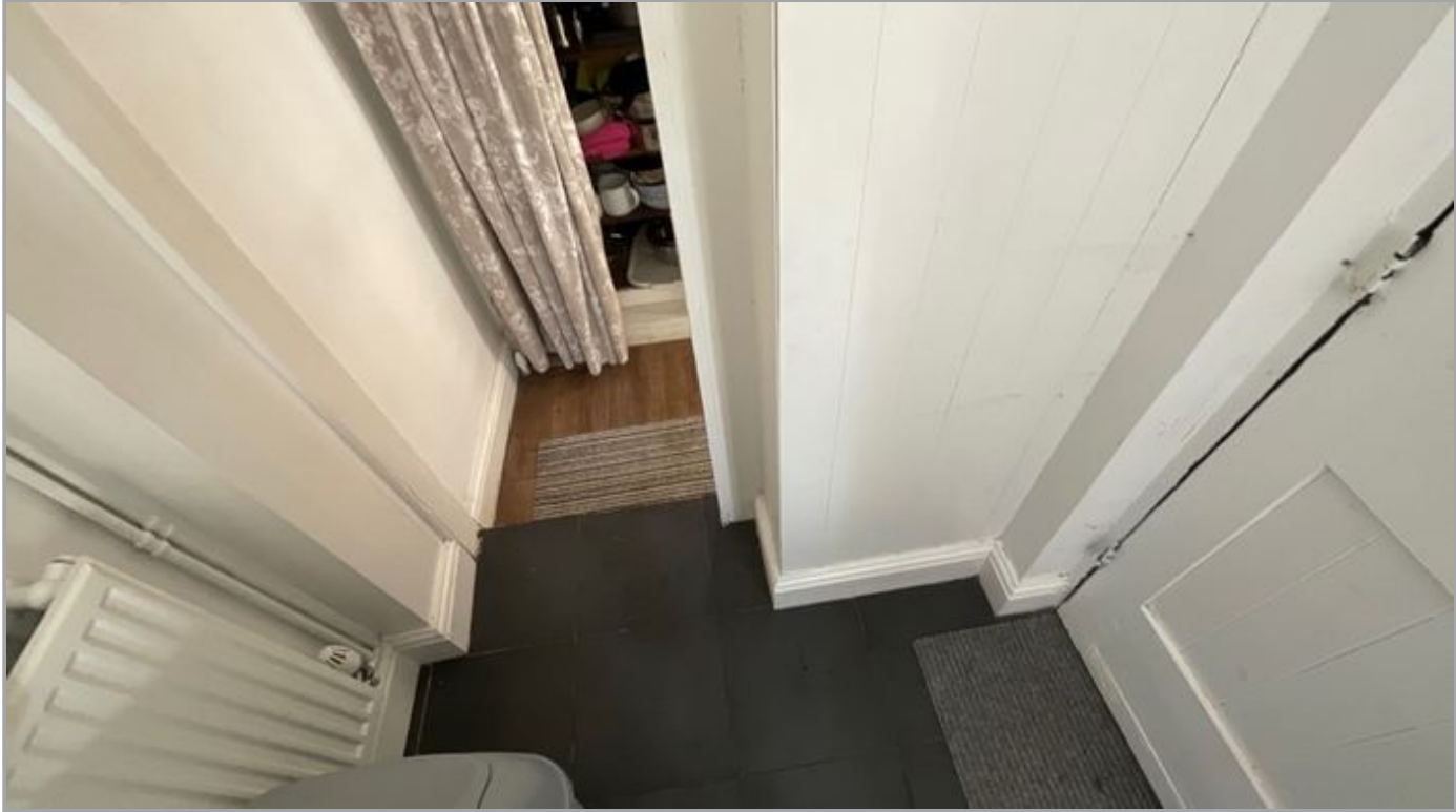
Wall Covered - See Limitations To Inspection
