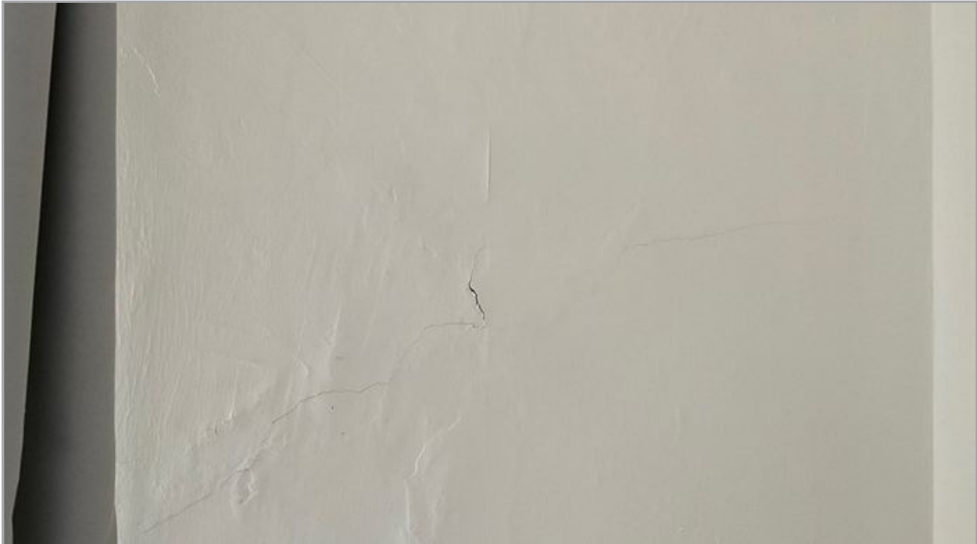
Shrinkage/De-bonding
