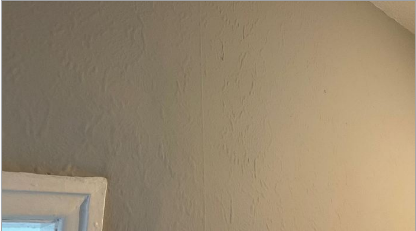
Wall Covered - See Limitations To Inspection
