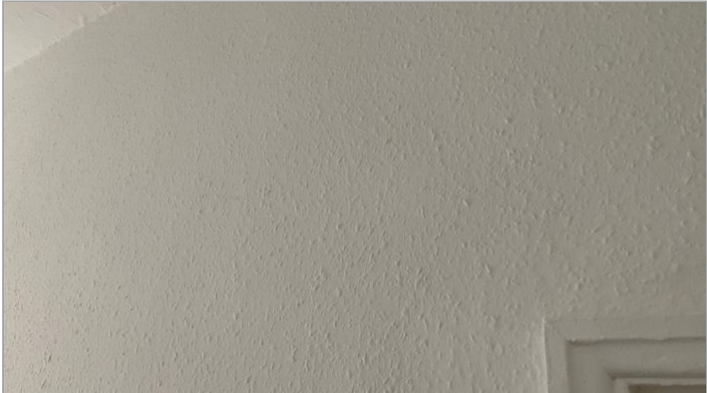
Wall Covered - See Limitations To Inspection
