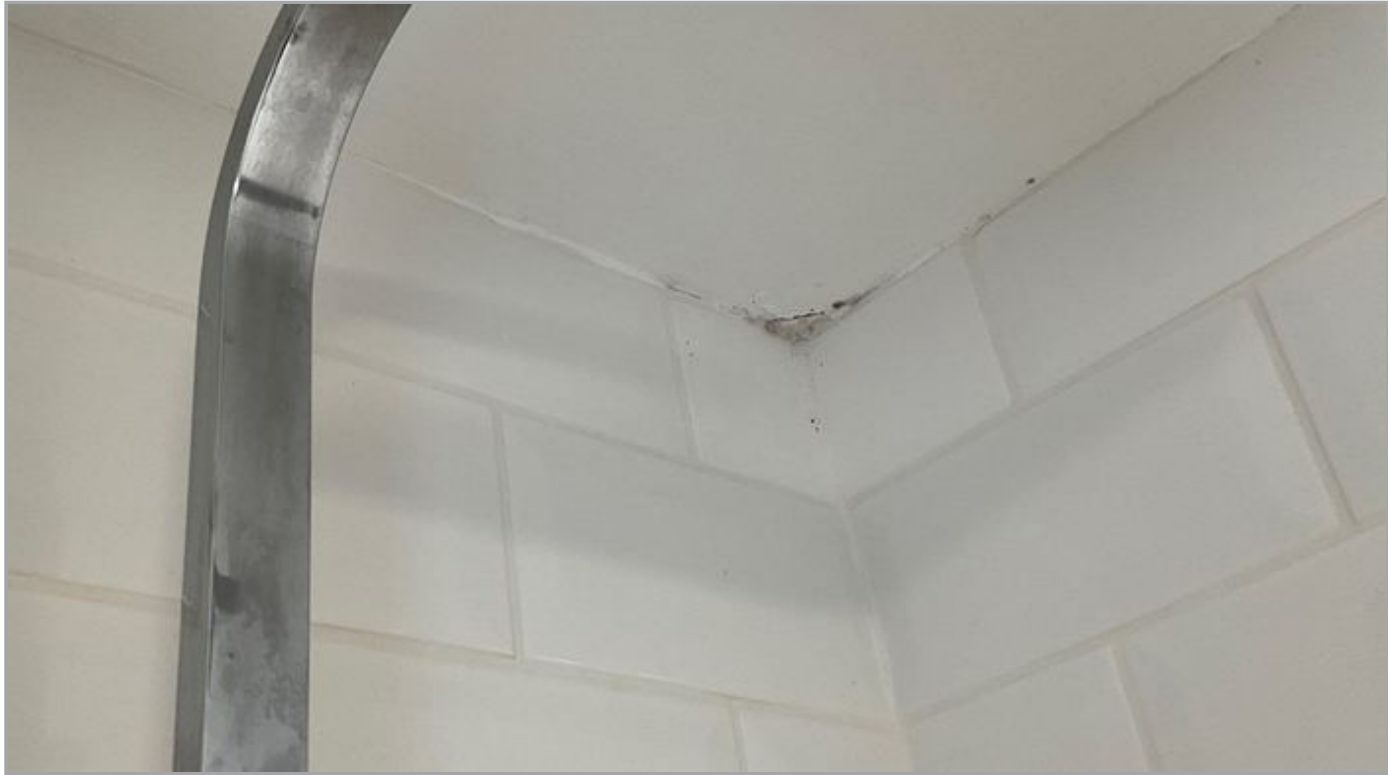
Condensation/Mould
