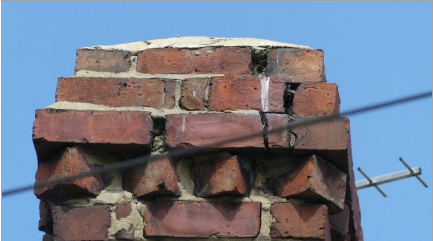
Eroding Pointing
