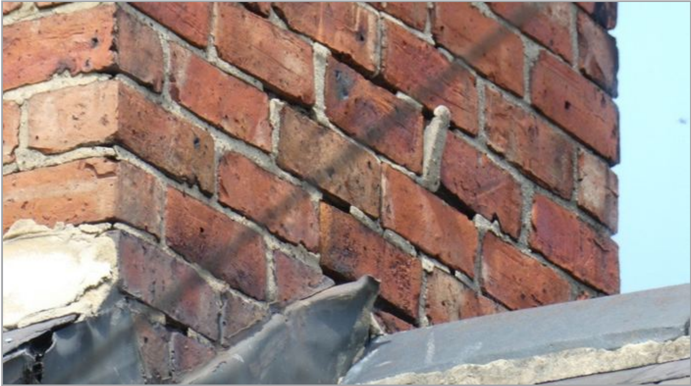
Eroding Pointing
