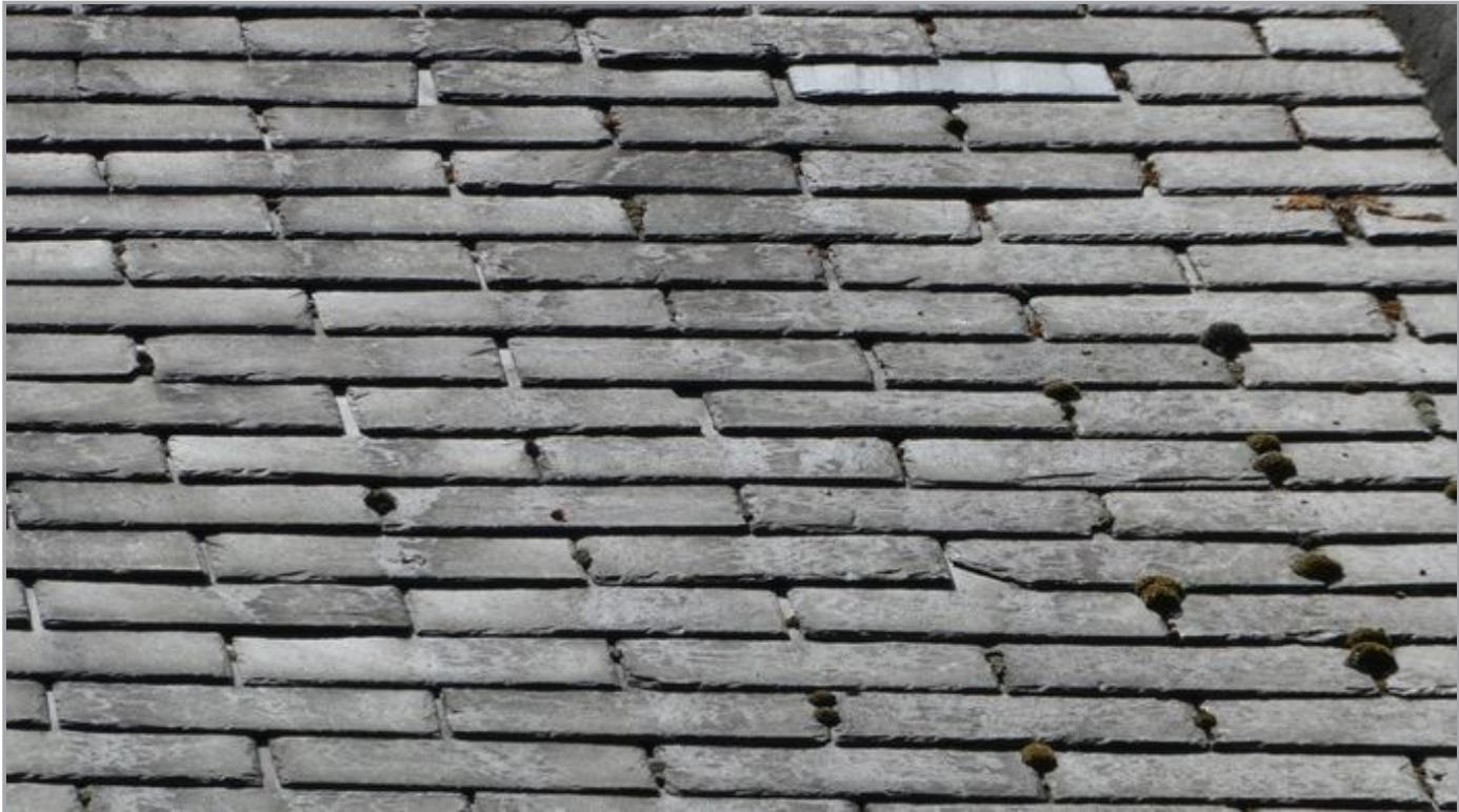
Lifted/Loose/Damaged Coverings
