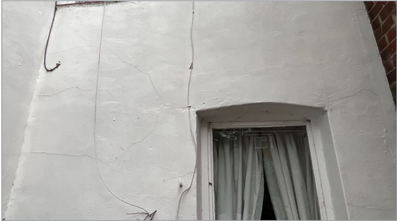
Render Cracking
