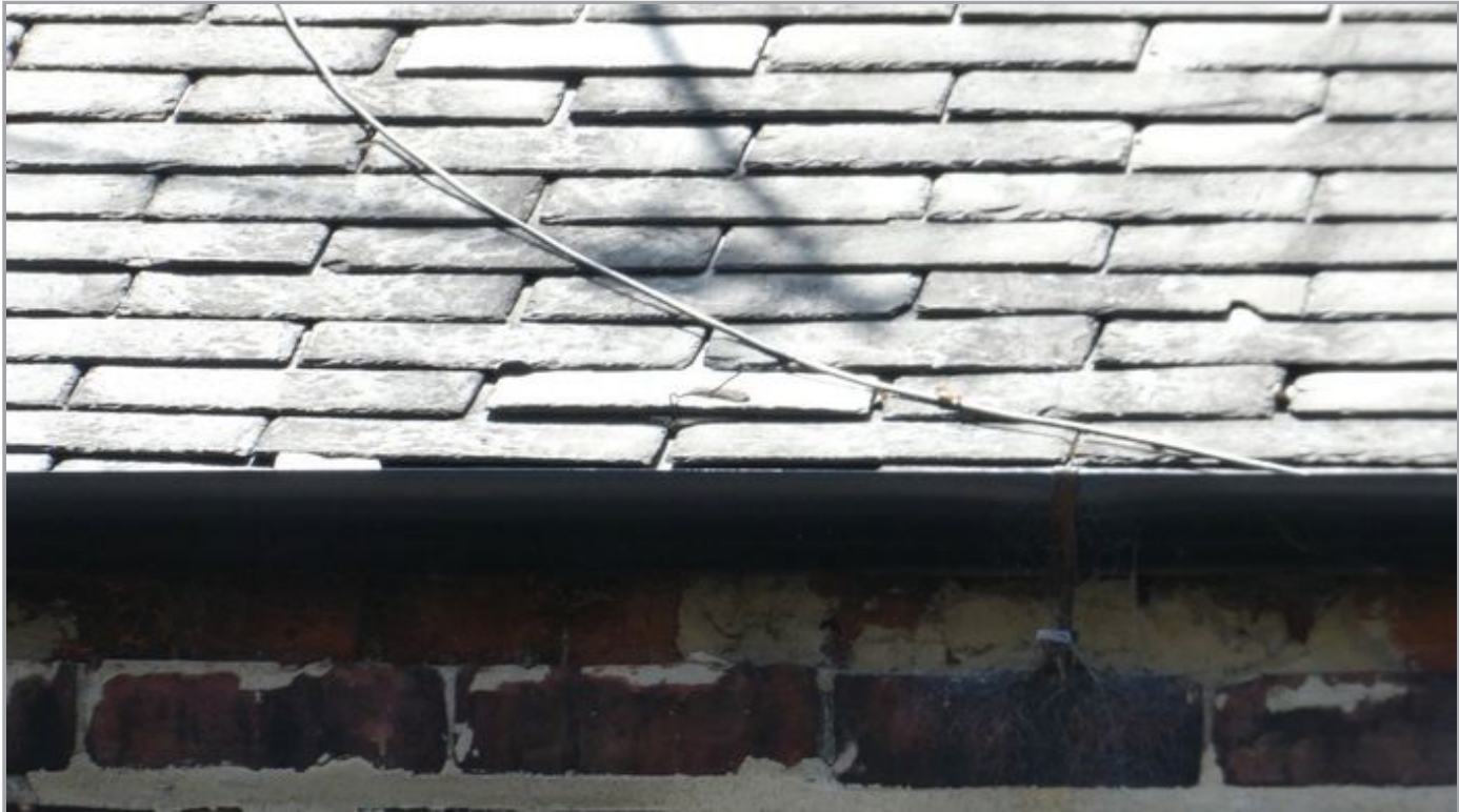
Lifted/Loose/Damaged Coverings
