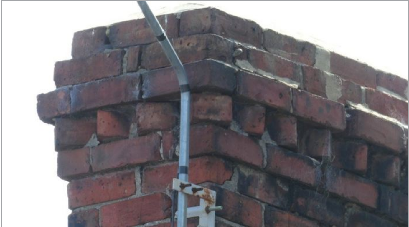
Eroding Pointing
