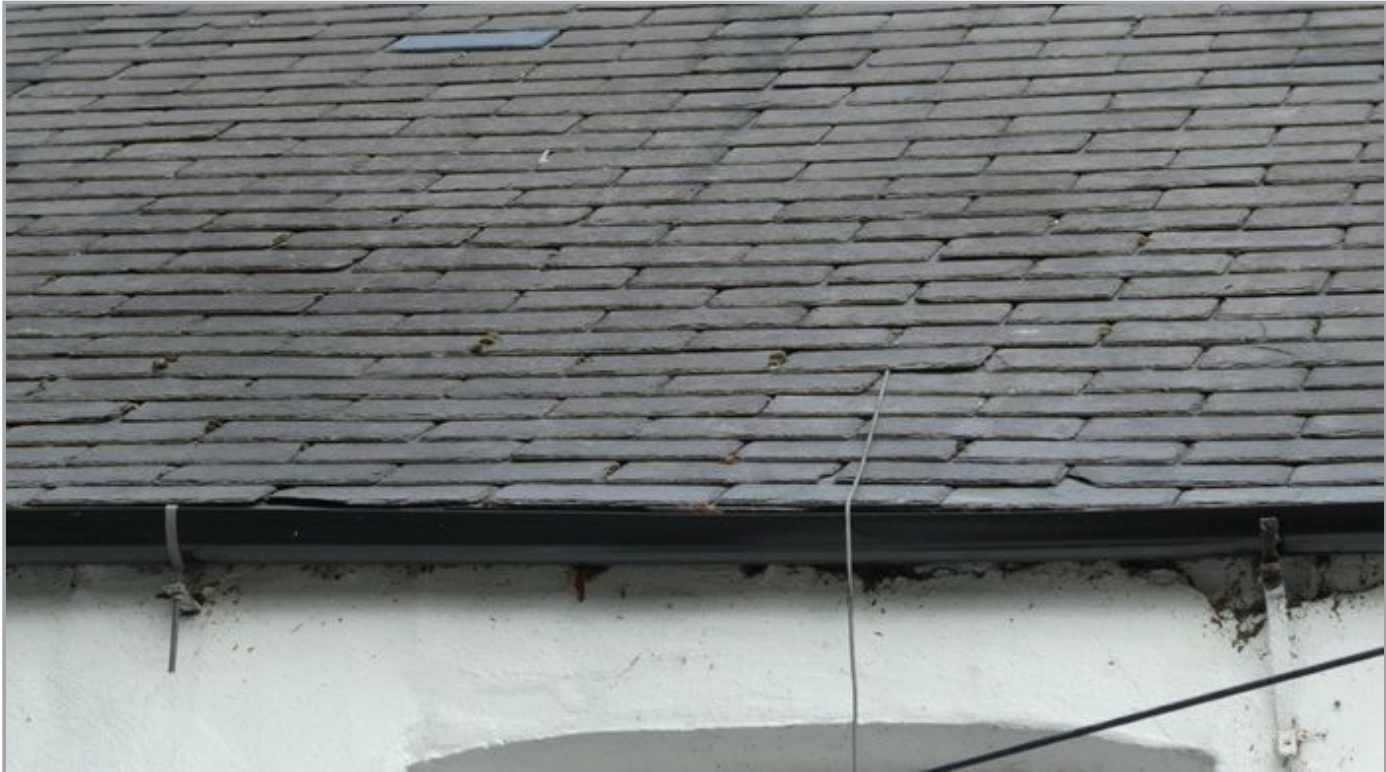
Lifted/Loose/Damaged Coverings
