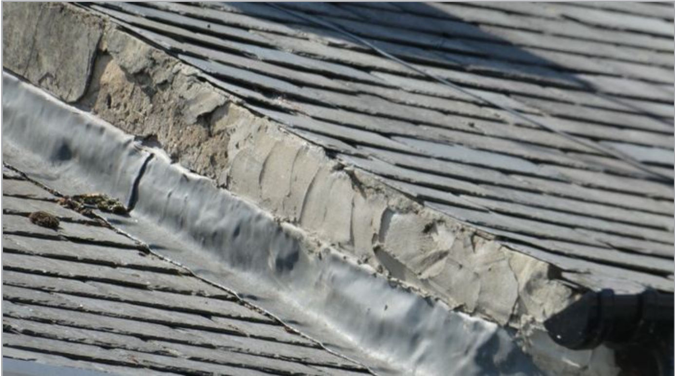
Inadequate Flashing
