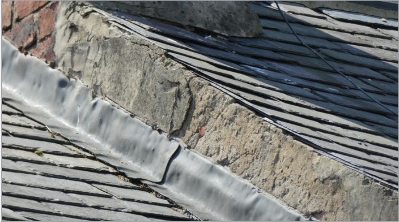
Inadequate Flashing
