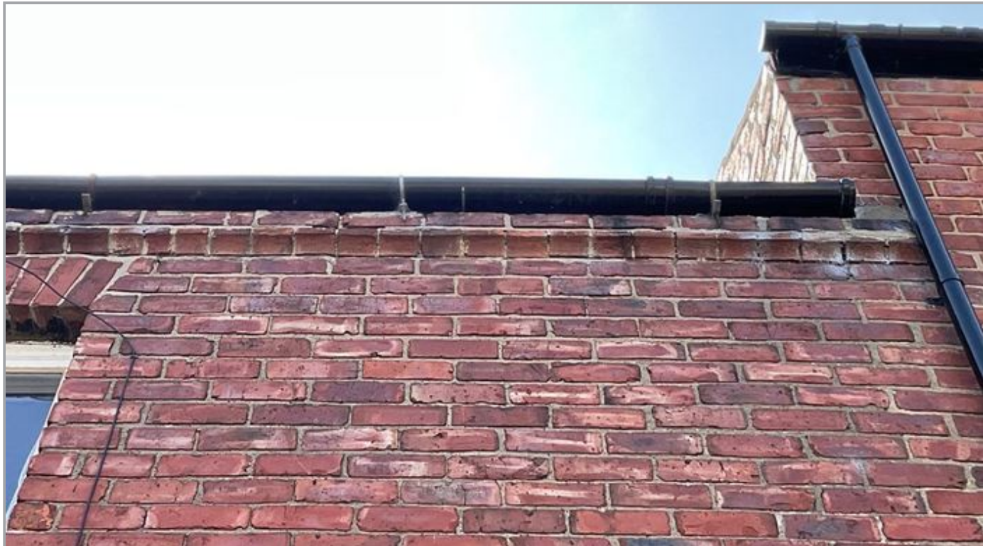
Eroding Pointing
