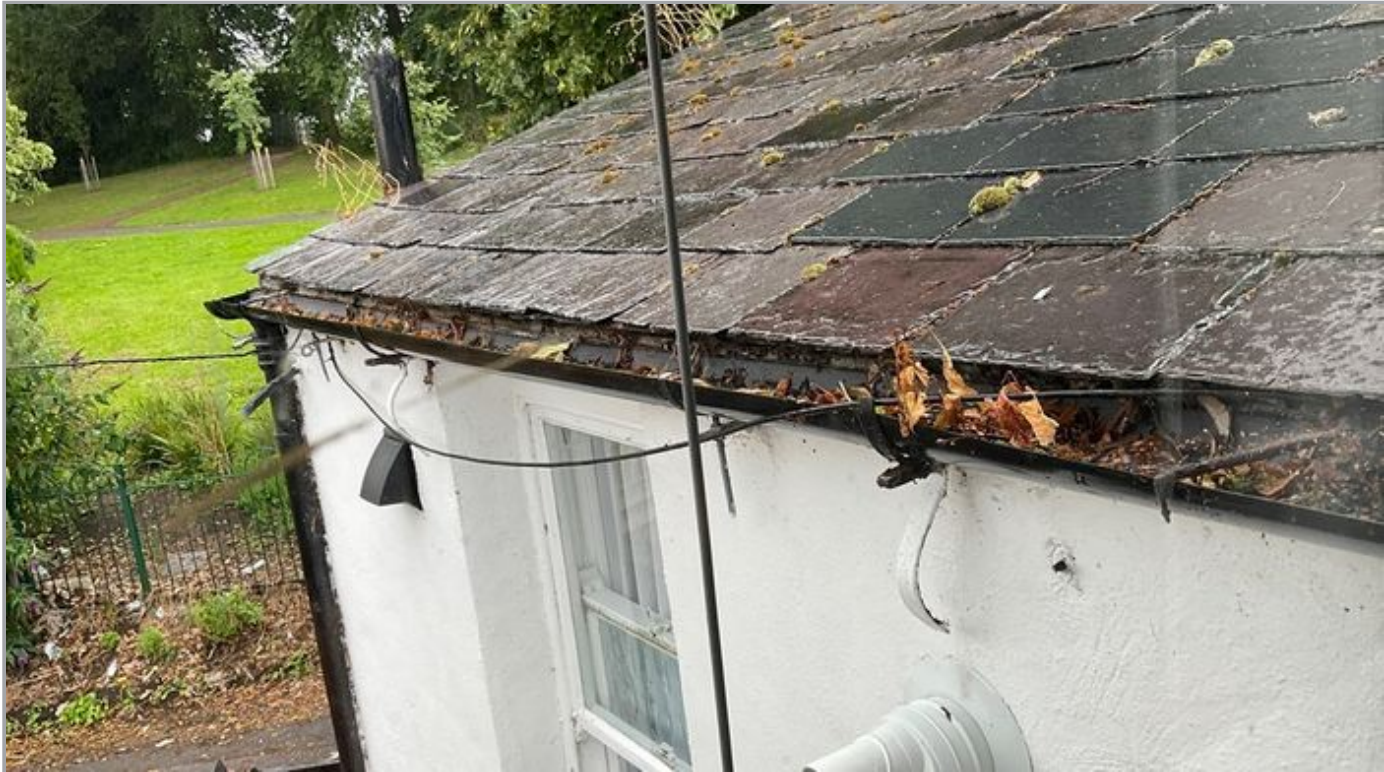
Blocked Guttering
