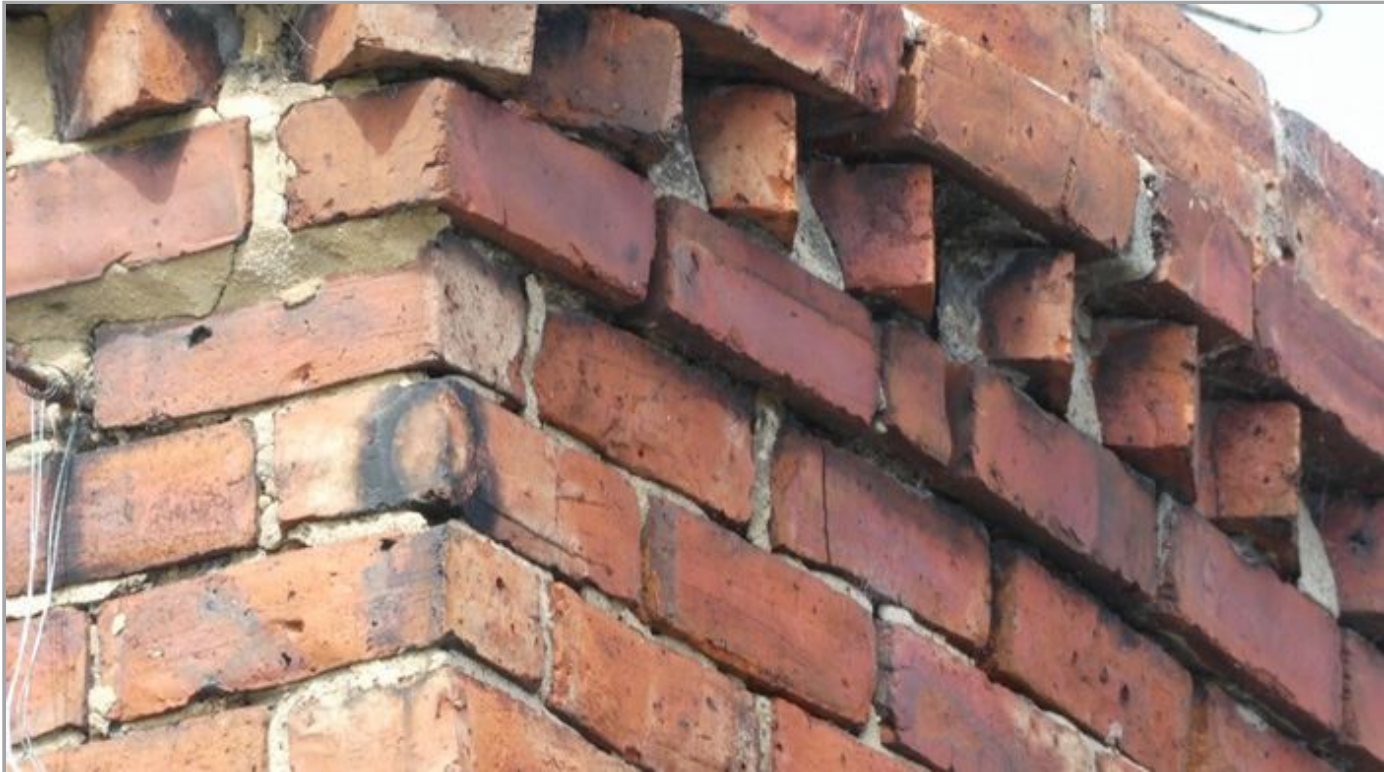
Eroding Pointing
