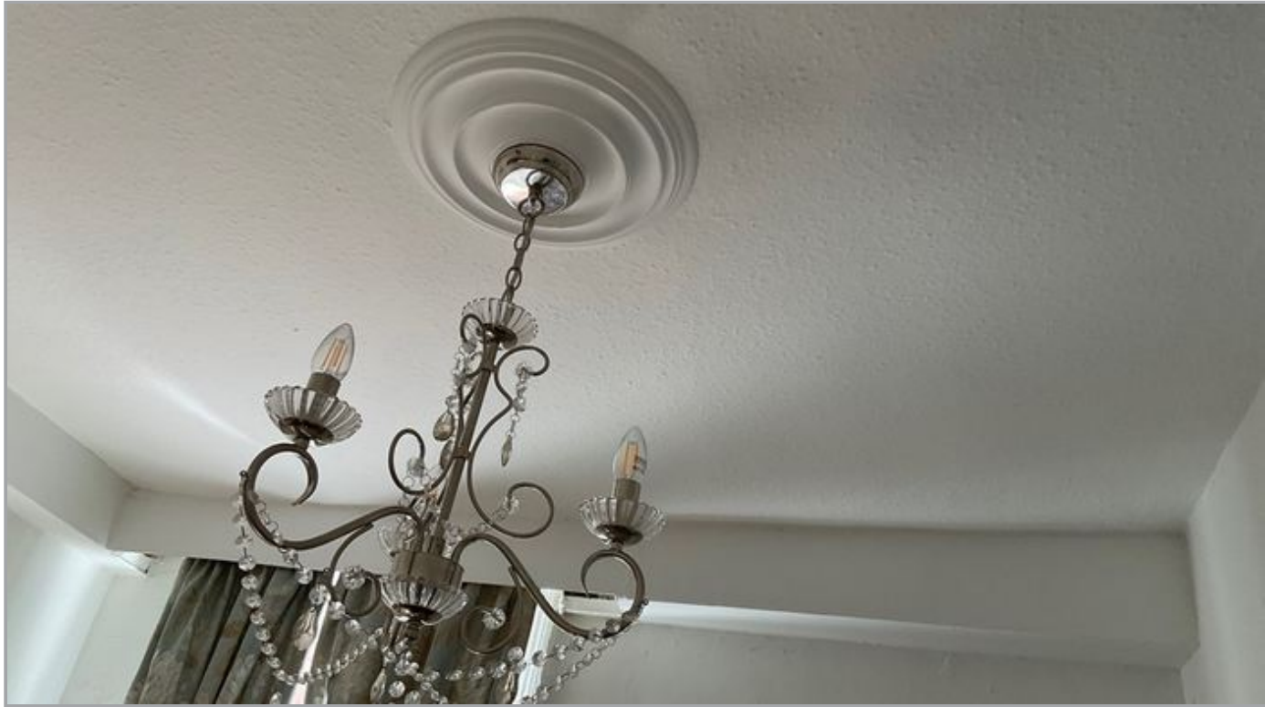
Ceiling Covered - See Limitations To Inspection
