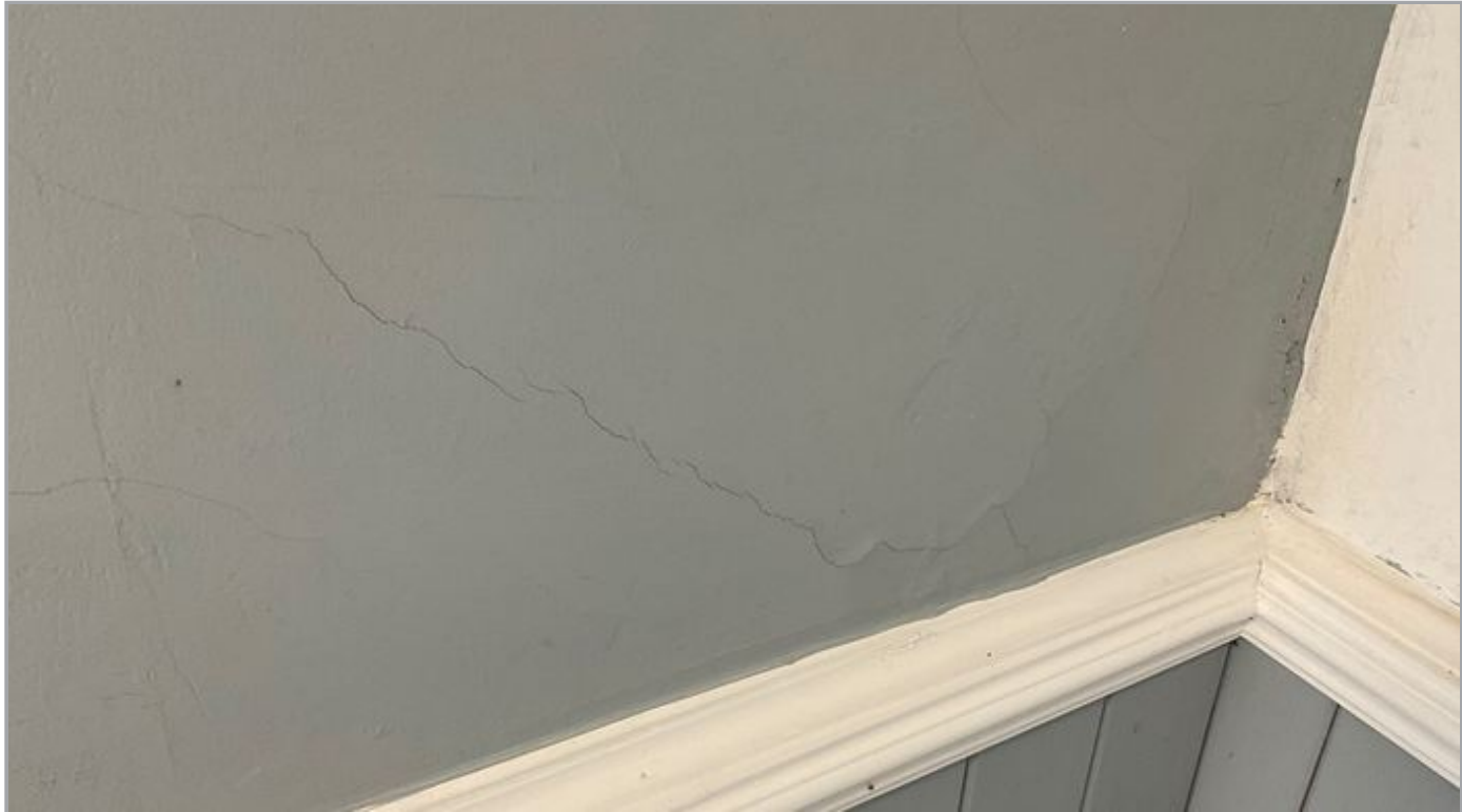
Shrinkage/De-bonding
