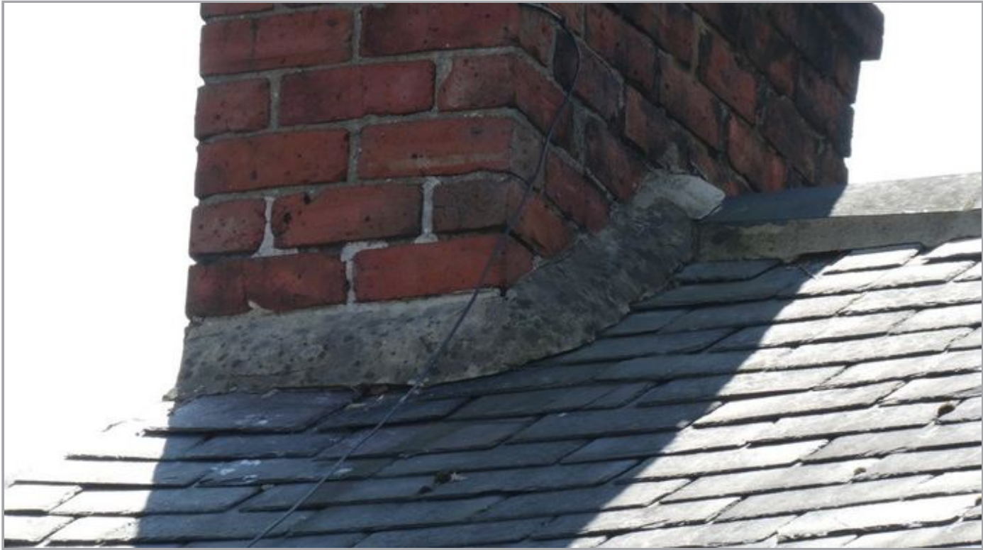
Inadequate Flashing
