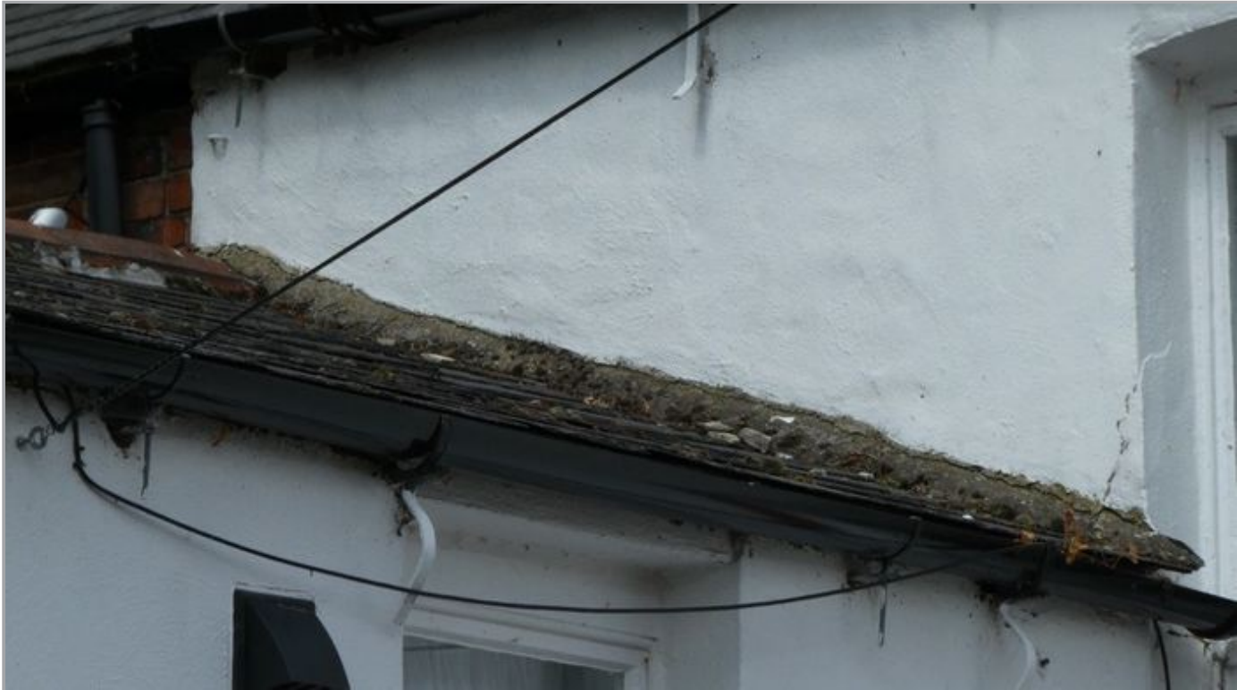
Inadequate Flashing
