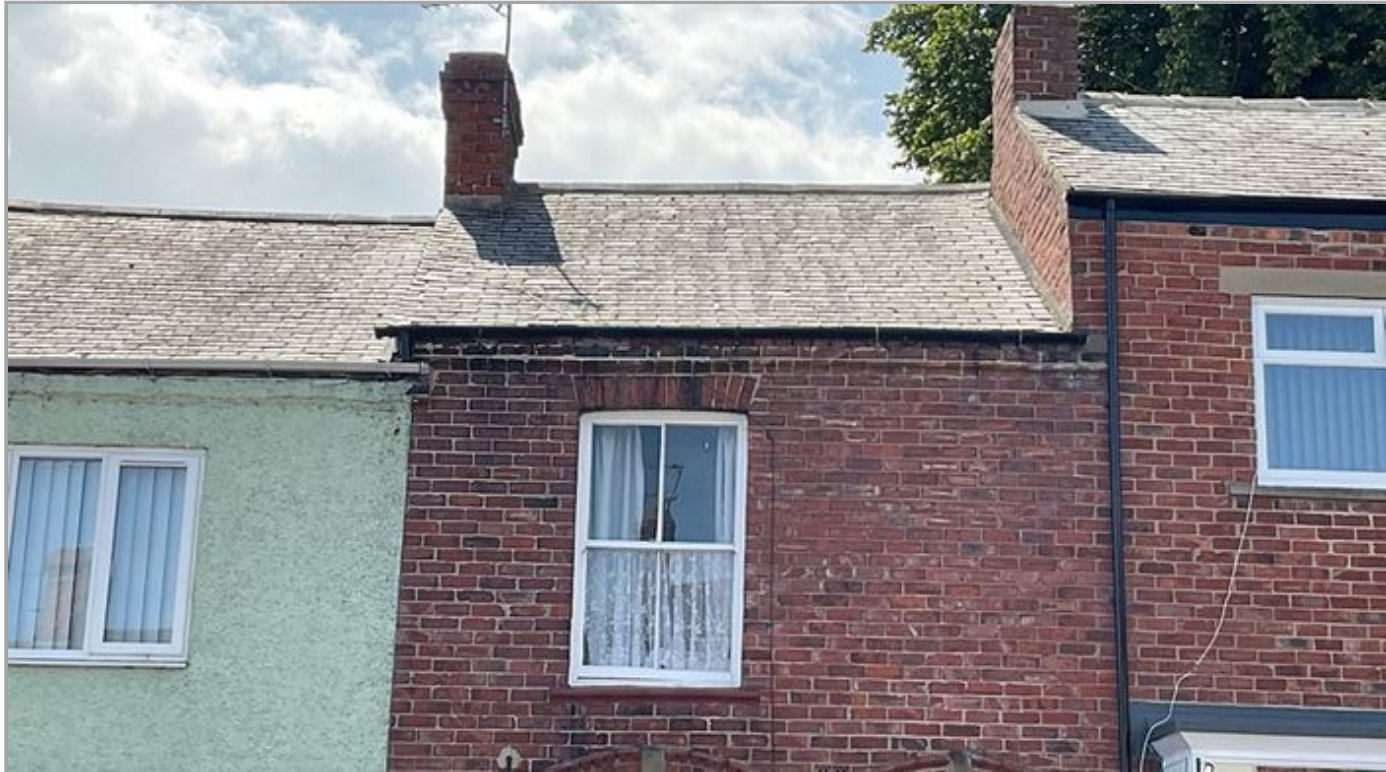
Misaligned Guttering
