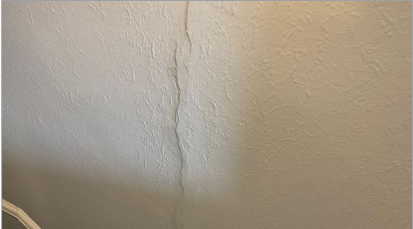
Wall Covered - See Limitations To Inspection
