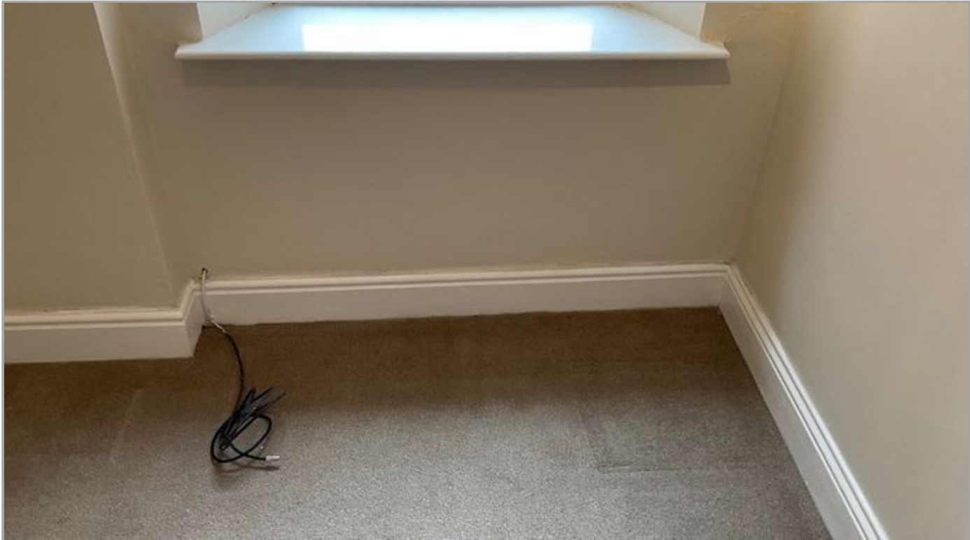
Springy Flooring Rear Bedroom
