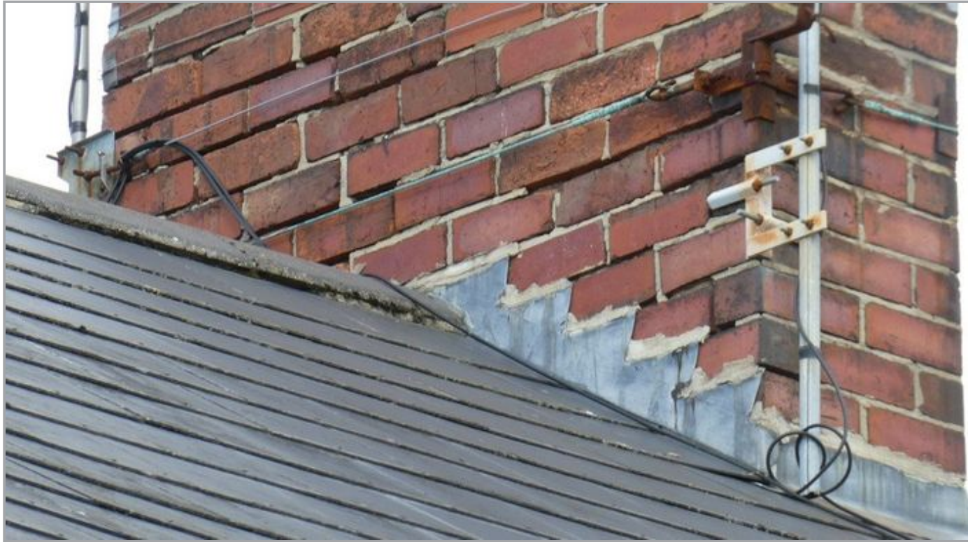
Eroding Pointing
