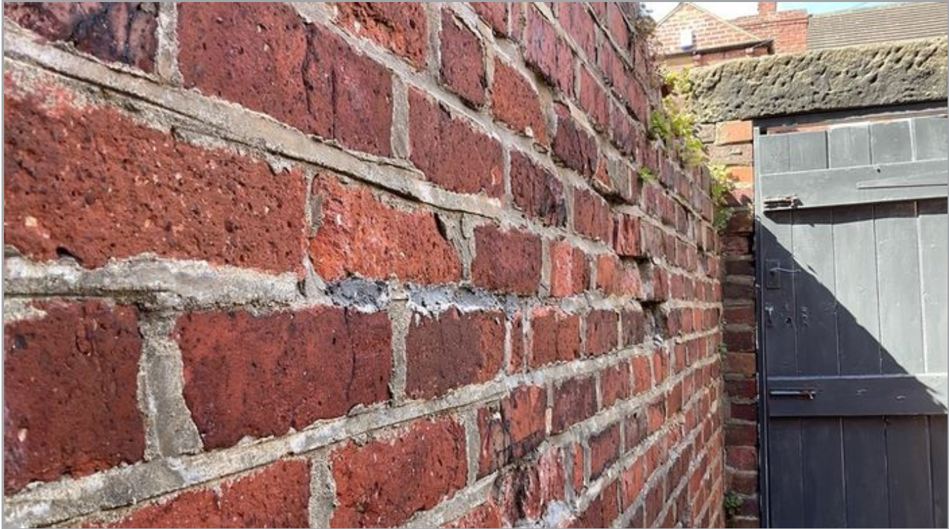
Pointing/Spalling
