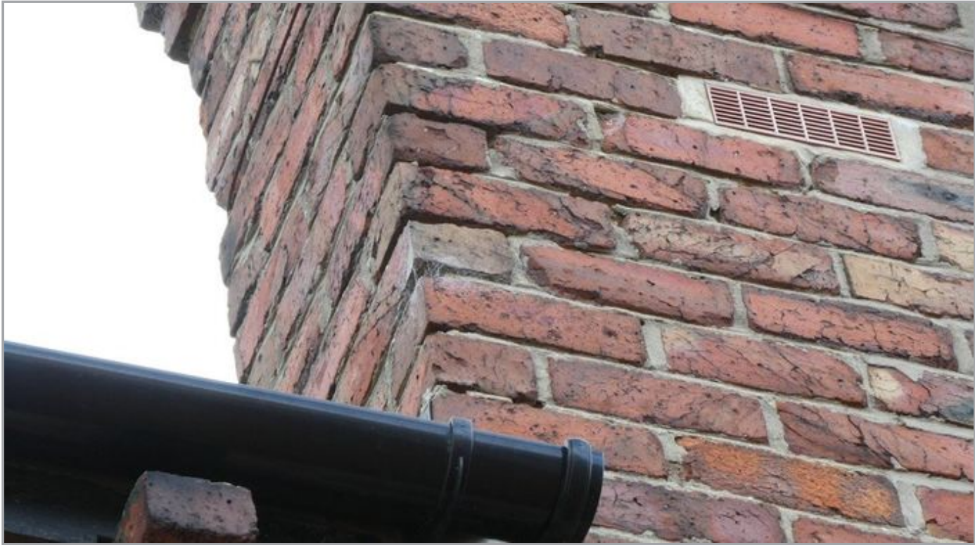
Eroding Pointing
