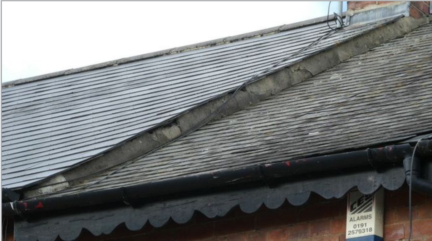
Inadequate Junction
