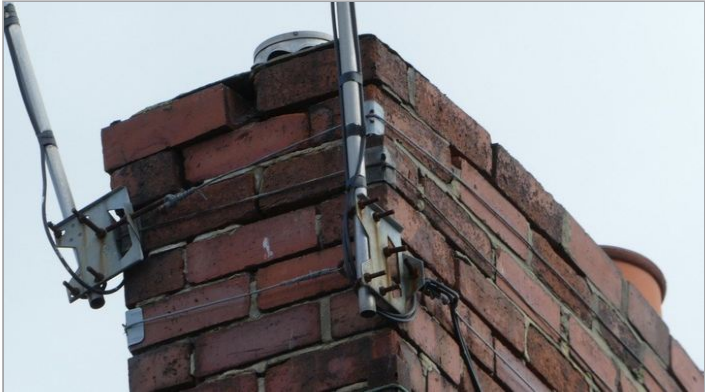
Eroding Pointing
