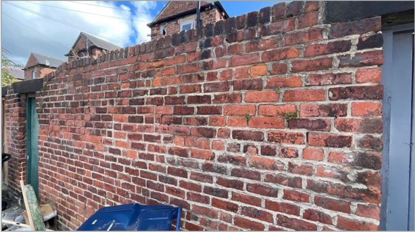
Pointing/Spalling
