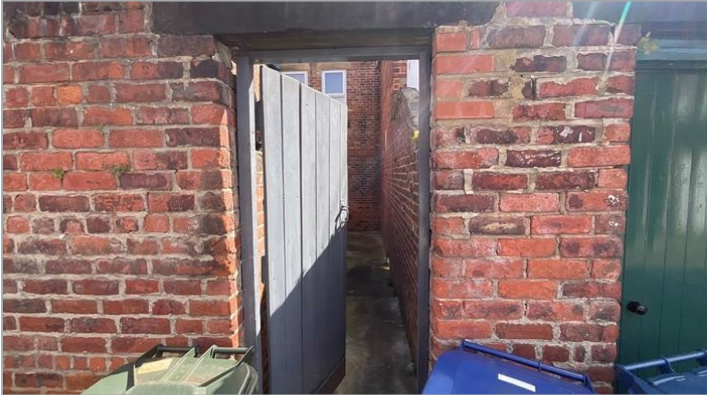
Pointing/Spalling
