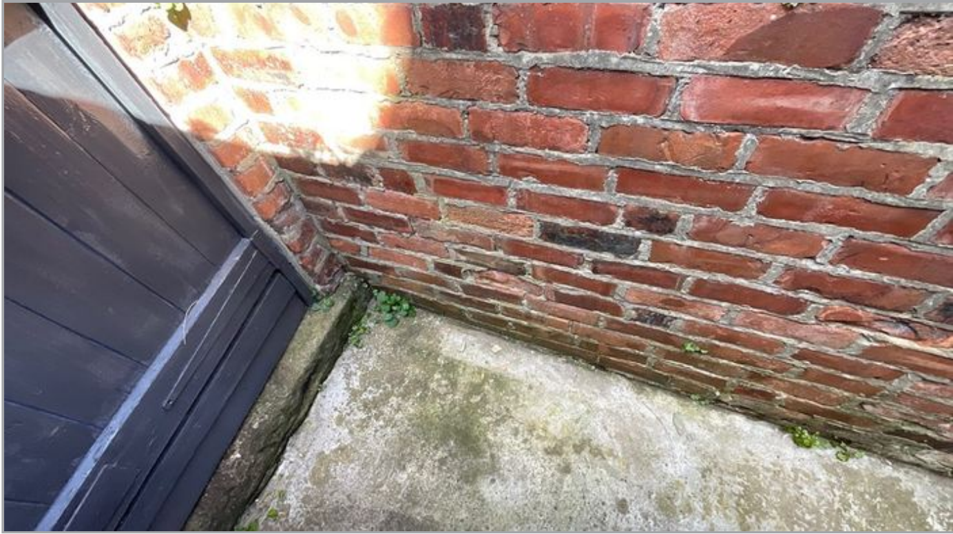
Pointing/Spalling
