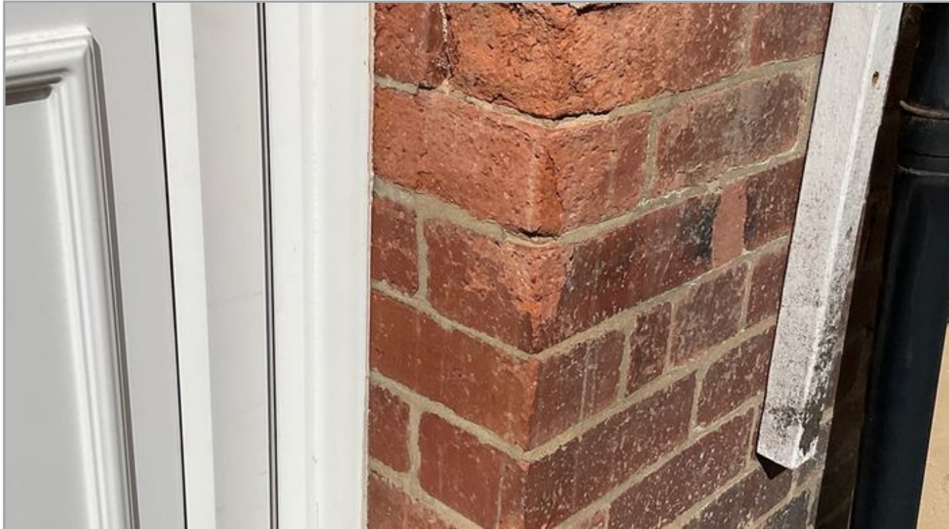
Spalling Brickwork
