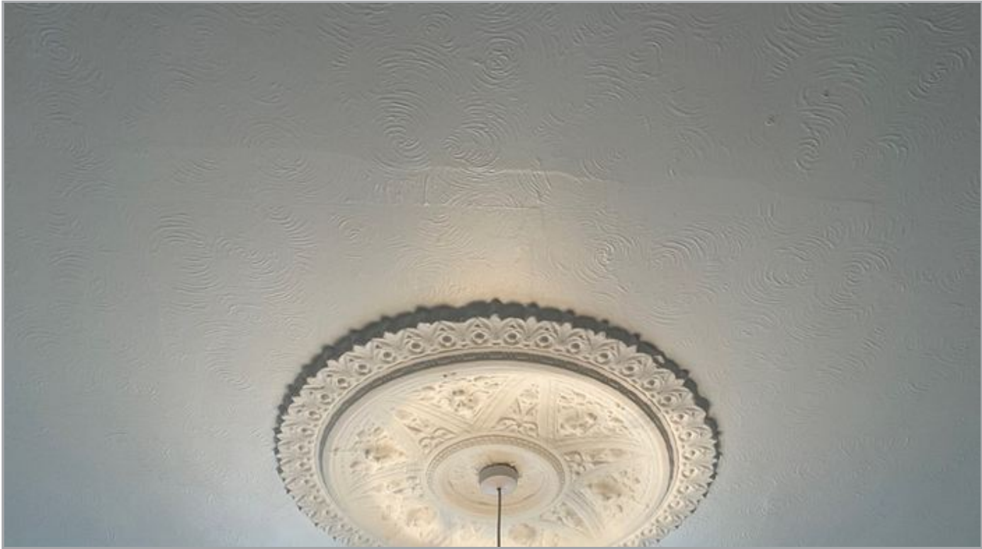
Ceiling Covered - See Limitations To Inspection
