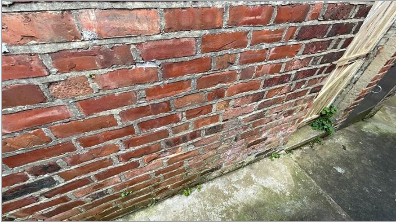
Pointing/Spalling
