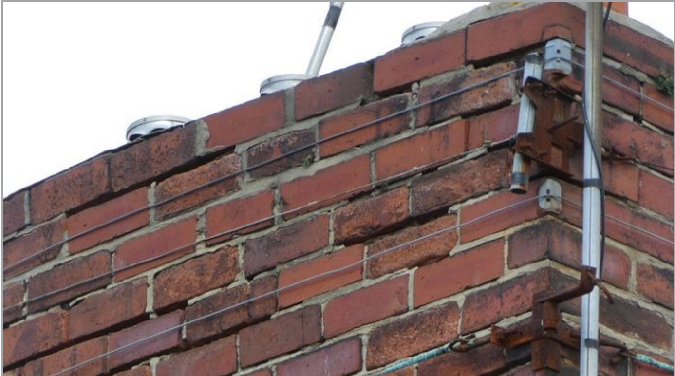
Eroding Pointing
