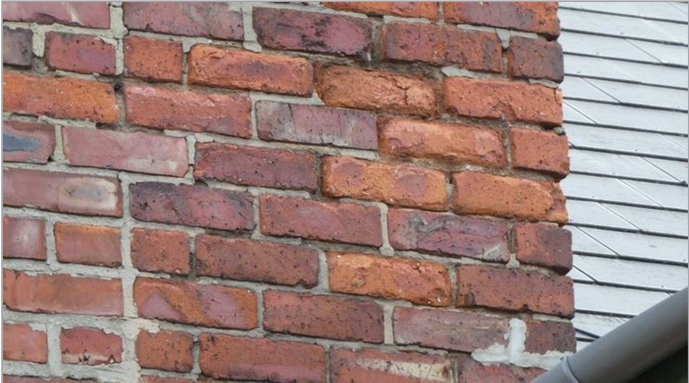
Eroding Pointing
