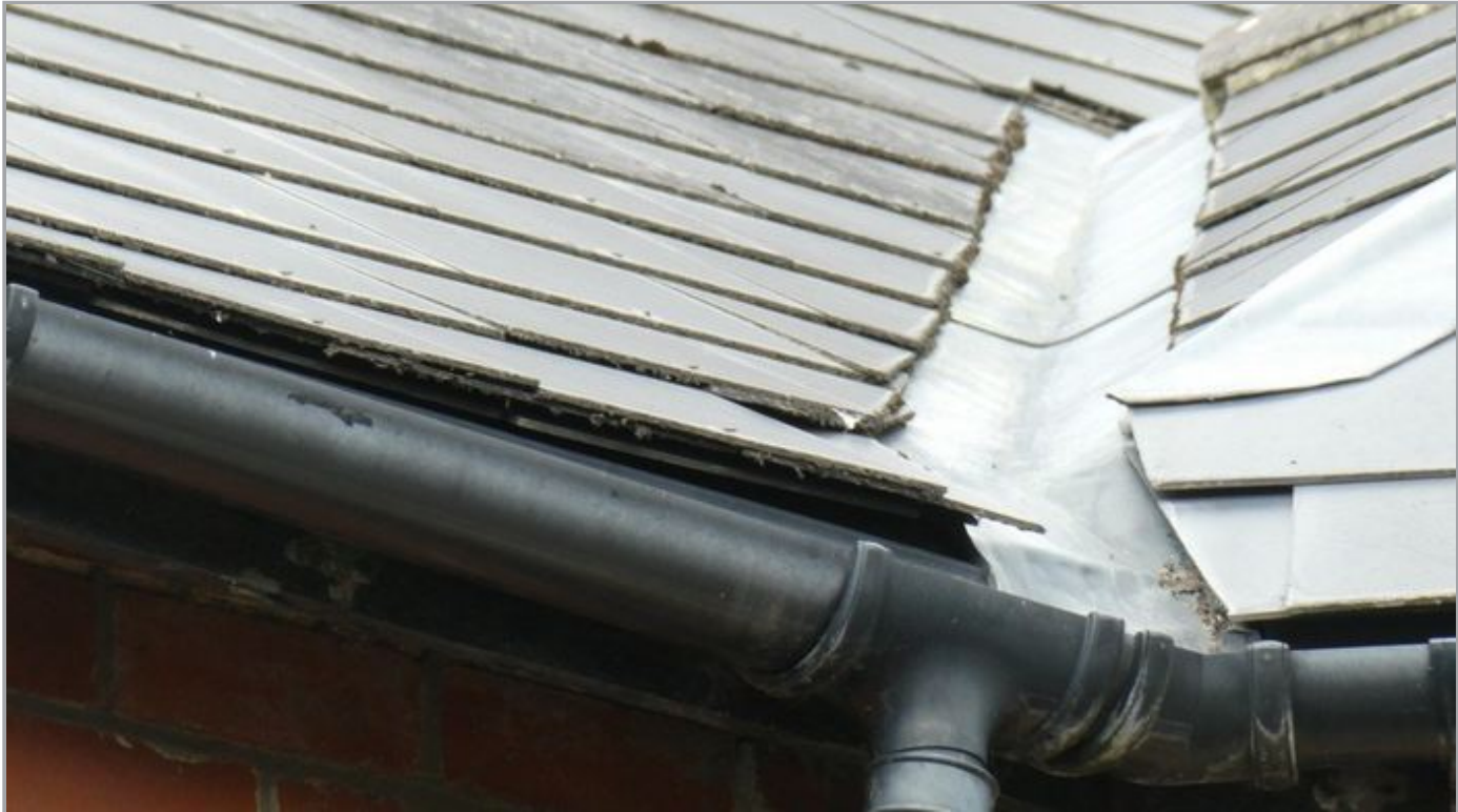
Valley Gutter No Blockages
