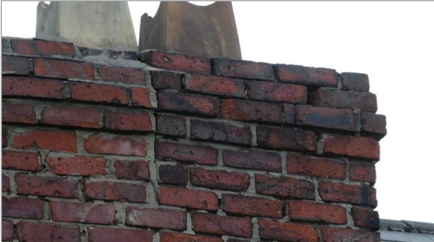
Eroding Pointing
