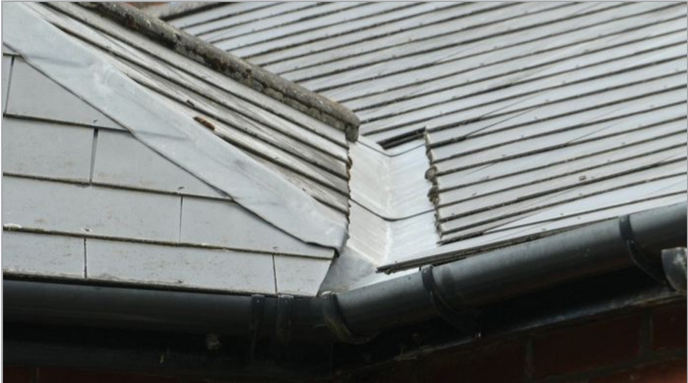
Valley Gutter No Blockages
