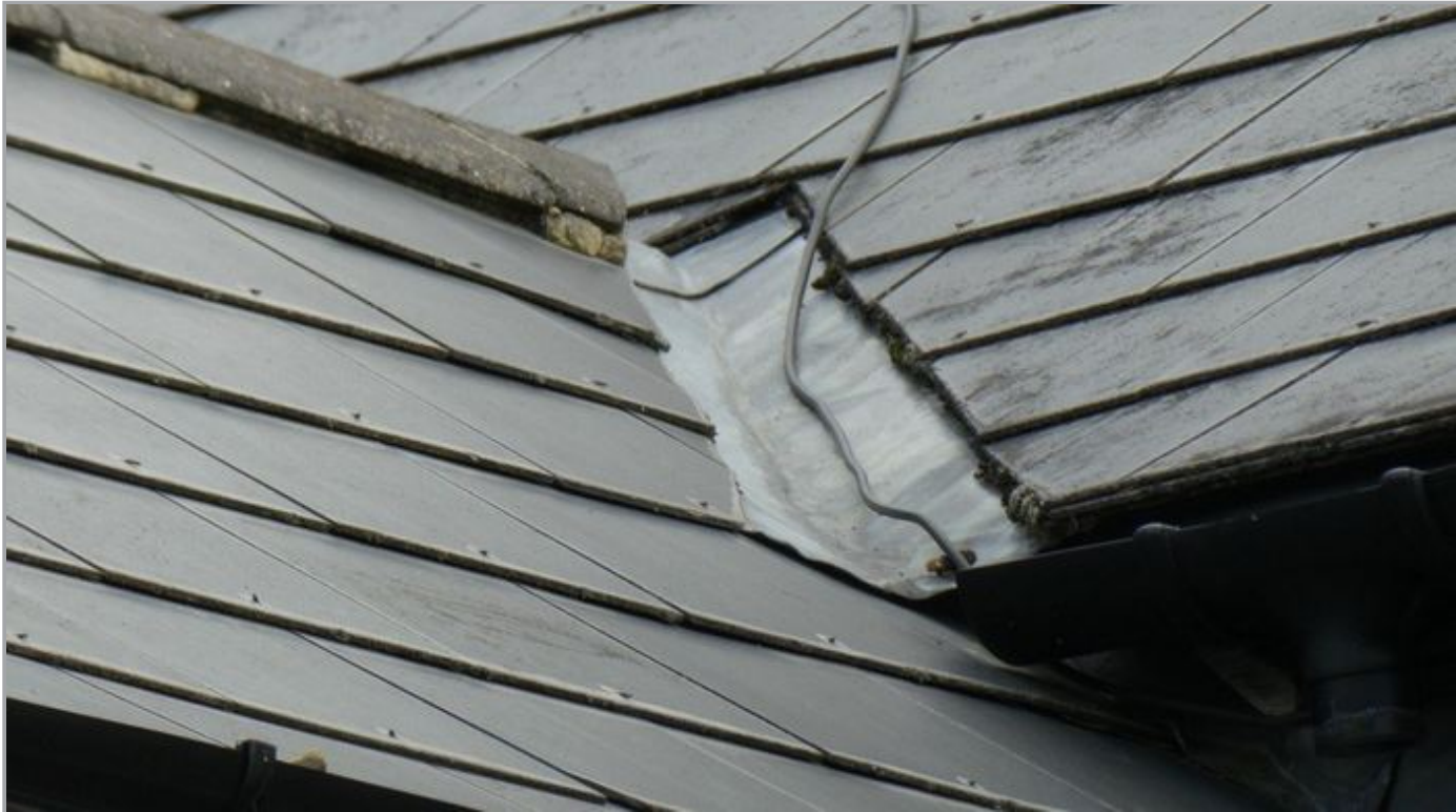
Valley Gutter No Blockages
