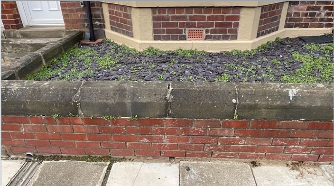
Inadequate Ventilation
