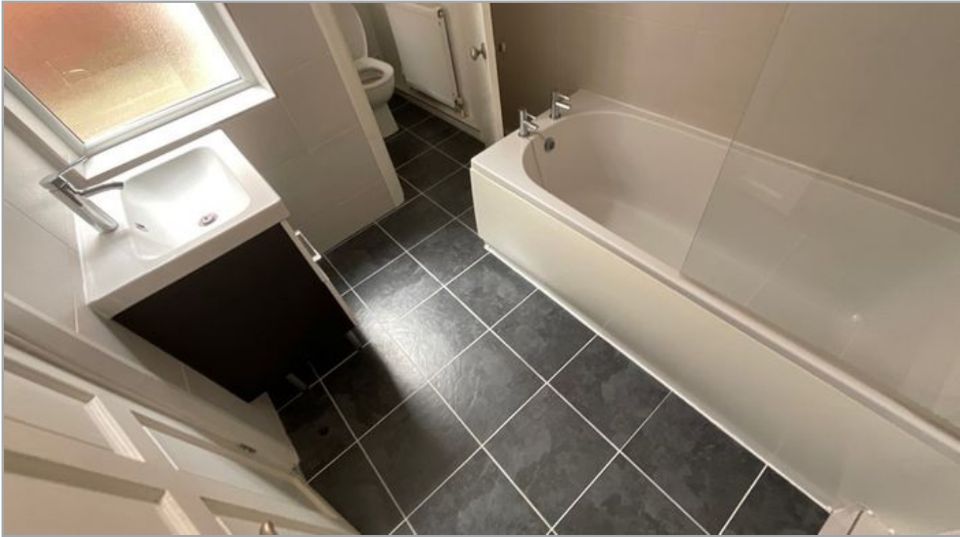
Wall Covered - See Limitations To Inspection
