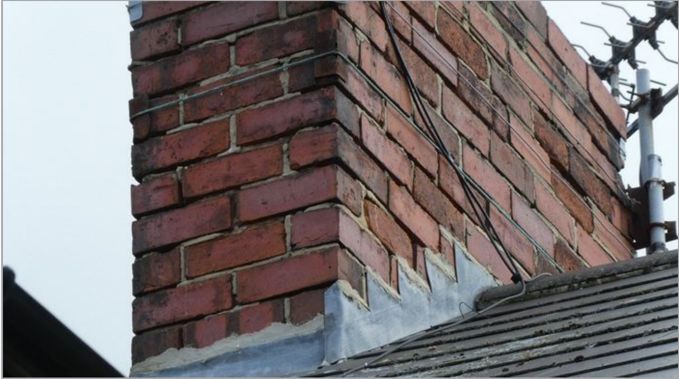
Eroding Pointing
