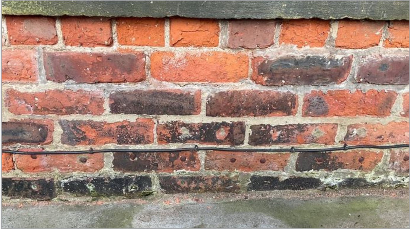
Spalling Brickwork
